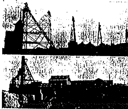
Figs. 5 and 6—The Granite Mountain headframe is seen above. Below is the surface plant at the Speculator shaft.
